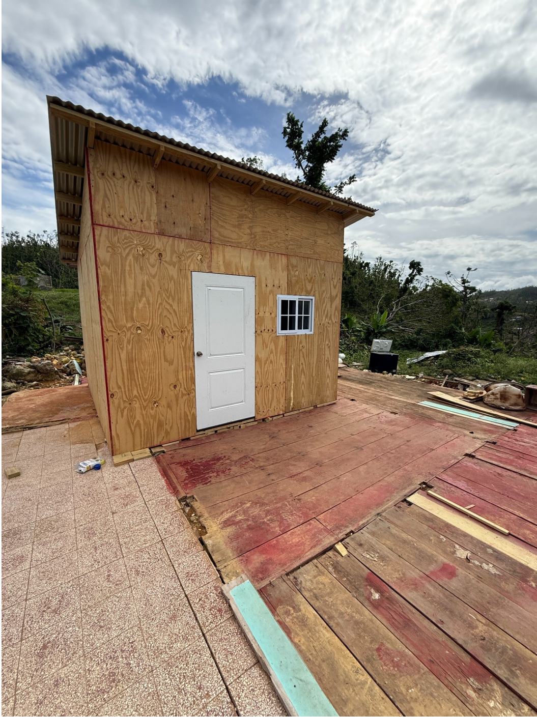
A newly constructed 12x12 home built during Rooted Legacy's Jamaica relief mission, helping provide shelter and restoration assistance to families impacted by the storm.
